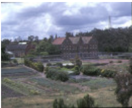
1 former convent of the good shepherd clarke street abbotsford view of property nov1981 etc.
