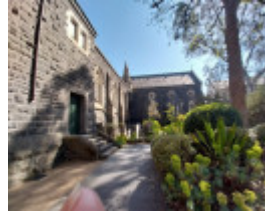
Convent Chapel view from south Oct 2024
