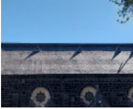
Convent Chapel roof detail Oct 2024
