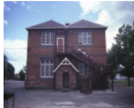
Primary School No. 1181, Bridport Street Albert Park, side entrance, Dec 1984
