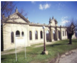
h00358 old hospital ruins church st beechworth view facade she project 2003
