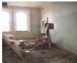
H1590 FORMER RUPANYUP RAILWAY STATION LHA 2015 7.JPG
