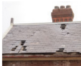
H1590 FORMER RUPANYUP RAILWAY STATION LHA 2015 4.JPG
