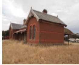
H1590 FORMER RUPANYUP RAILWAY STATION LHA 2015 1.JPG
