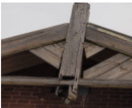
H1590 FORMER RUPANYUP RAILWAY STATION LHA 2015 5.JPG
