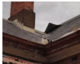
H1590 FORMER RUPANYUP RAILWAY STATION LHA 2015 6.JPG
