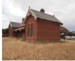
H1590 FORMER RUPANYUP RAILWAY STATION LHA 2015 1.JPG
