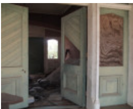
H1590 FORMER RUPANYUP RAILWAY STATION LHA 2015 8.JPG
