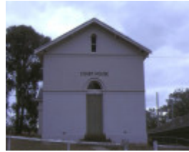
1 rushworth courthouse rushworth front elevation nov1984
