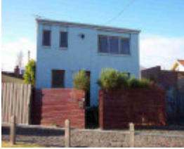
fitzroy north circle place fitzroy north circle place 5
