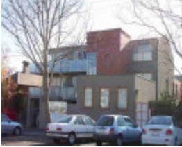
fitzroy north mckean street fitzroy north mckean street 137-149 unit 1
