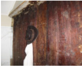
26 Finch slab wall of kitchen
