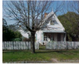
1 residence 26 finch street beechworth
