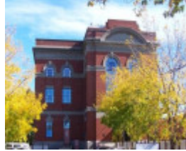
Victorian Railways DC Substation
