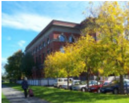
Victorian Railways DC Substation
