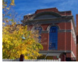
Victorian Railways DC Substation
