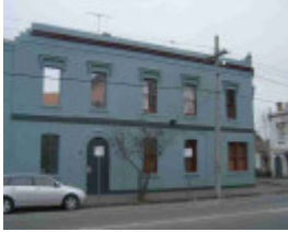
fitzroy north reid street fitzroy north reid street 62 unit 3
