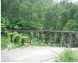
RAIL BRIDGE SOHE 2008
