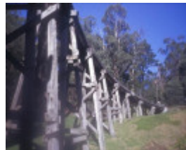
h01439 rail bridge over monbulk creek selby towards menzies creek she project she
