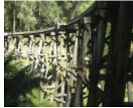
1 railway trestle bridge over monbulk creek selby side elevation apr1997
