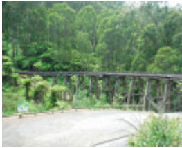
RAIL BRIDGE SOHE 2008
