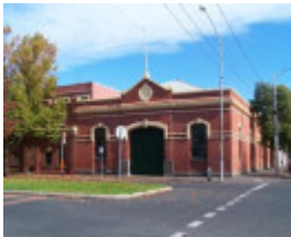
Cable Tram Engine House
