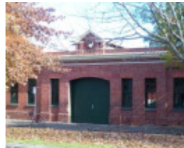
Cable Tram Engine House
