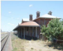
SERVICETON RAILWAY STATION SOHE 2008
