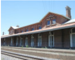
SERVICETON RAILWAY STATION SOHE 2008
