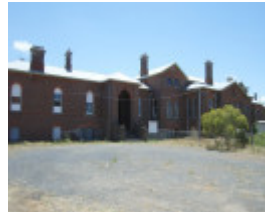
SERVICETON RAILWAY STATION SOHE 2008
