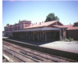
1 seymour railway station station street seymour platform view dec 1983
