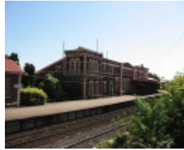
Seymour RWS Railway Building Road Side February 2002
