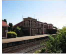
Seymour RWS Railway Building Road Side February 2002
