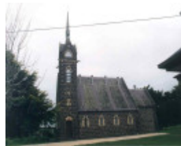
1 st andrews presbyterian church skipton side elevation 1995
