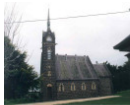
1 st andrews presbyterian church skipton side elevation 1995
