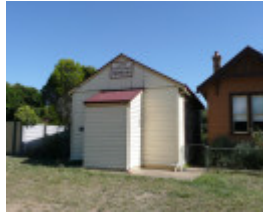
SKIPTON COURT HOUSE SOHE 2008
