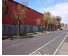
Former Coal Shed.JPG
