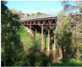
Victoria Street Bridge
