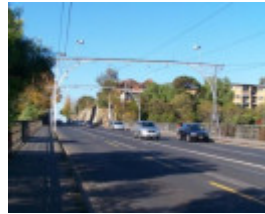
Victoria Street Bridge
