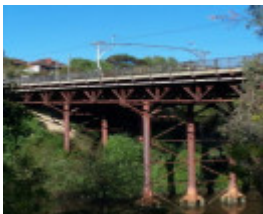
Victoria Street Bridge
