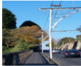
Victoria Street Bridge
