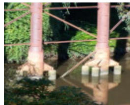
Victoria Street Bridge
