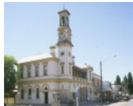
beechworth post office ford street beechworth side view
