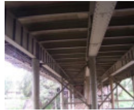
Yarra River Bridge
