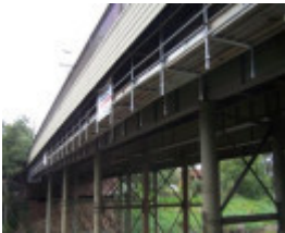
Yarra River Bridge
