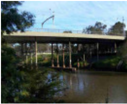
Yarra River Bridge
