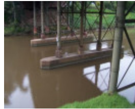
Yarra River Bridge
