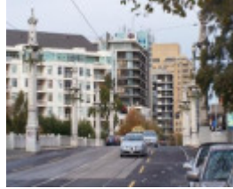
Church Street Bridge
