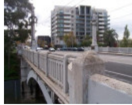
Church Street Bridge
