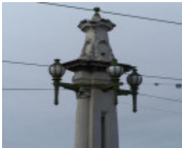
Church Street Bridge
