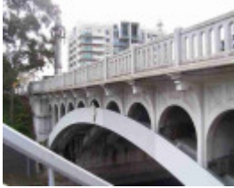
Church Street Bridge
