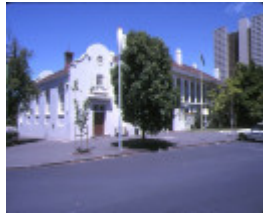
1 south melbourne court house & police station bank street south melbourne front view
