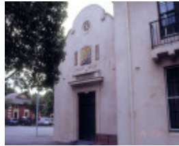
h01486 south melbourne court house and police station entry she project 2004
