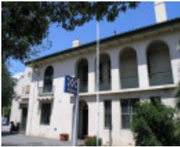
SOUTH MELBOURNE COURT HOUSE AND POLICE STATION SOHE 2008
