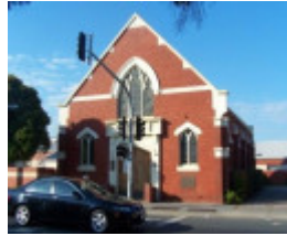
Burnley Uniting (former Presbyterian) Church
