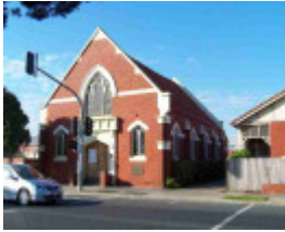
Burnley Uniting (former Presbyterian) Church
