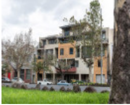
Millennium apartments facade 140 Queens Road Fitzroy North
