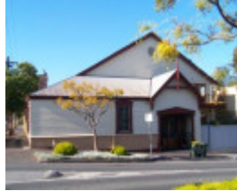
Richmond Orderly Room
