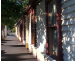
Richmond Orderly Room
