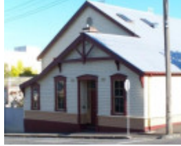
Richmond Orderly Room
