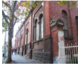
Melbourne Tramway and Omnibus Company Engine House
