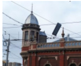
Melbourne Tramway and Omnibus Company Engine House
