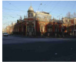
Melbourne Tramway and Omnibus Company Engine House
