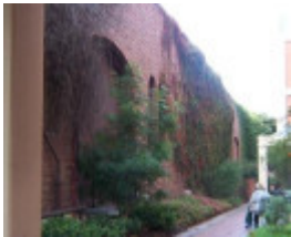
Melbourne Tramway and Omnibus Company Engine House
