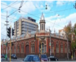
Melbourne Tramway and Omnibus Company Engine House
