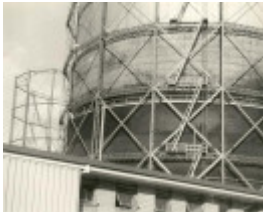
former gasometer alexandra parade 1975.jpg
