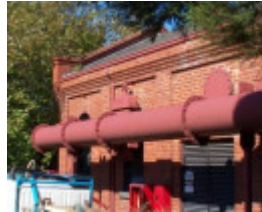
Fitzroy Gas Works Valve House
