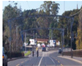
Ornamental tram poles
