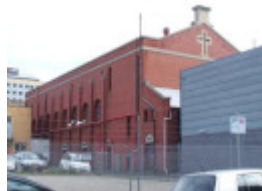
Cathedral Hall view from Young St
