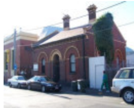
Gas Inspector's Residence
