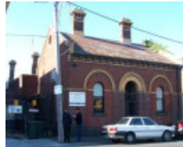
Gas Inspector's Residence
