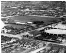
Image showing the gasometer in Gleadell Street
