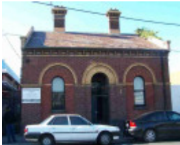
Gas Inspector's Residence
