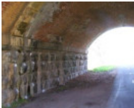
Hawthorn Railway Bridge
