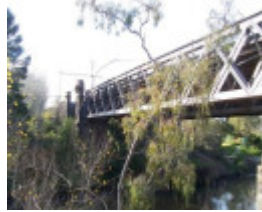
Hawthorn Railway Bridge
