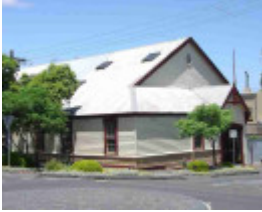
Richmond Orderly Room - 24 Gipps Street
