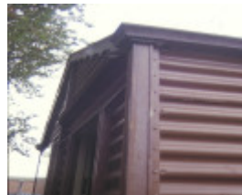
Abercrombie House 399 Coventry St Sth Melbourne Abercrombie Bellhouse Side Detail Jul 1999
