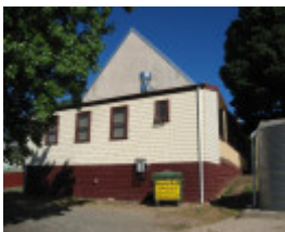
Church rear addition
