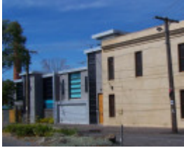
clifton hill wellington street clifton hill wellington street 432 rear
