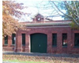
Cable Tram Engine House
