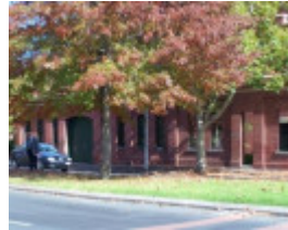
Cable Tram Engine House
