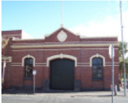
Cable Tram Engine House - 440 Park Street
