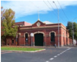
Cable Tram Engine House
