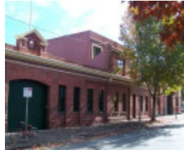
Cable Tram Engine House
