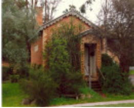
Former CBA Bank 810 Main Rd Eltham Colour 1 - Shire of Eltham Heritage Study 1992
