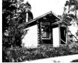
205 - Former CBA Bank 810 Main Rd Eltham 02 - 1949? photograph showing this building apparently still in use as a bank - note the signage, which includes gold leaf lettering on the window - Shire of Eltham Heritage Study 1992
