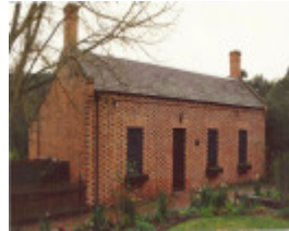
Shillinglaw Cottage Main Rd Eltham Colour 2 - Shire of Eltham Heritage Study 1992
