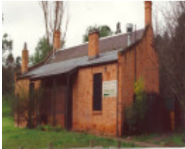
Shillinglaw Cottage Main Rd Eltham Colour 3 - Shire of Eltham Heritage Study 1992
