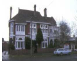
1 balladonia formerly arrou ferrars place south melbourne front view
