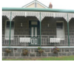
Athelston, 2025 Hamilton Highway, Murgheboluc viewed from east.
