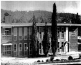
213 - 3 Pencil Pines at Council Offices Eltham - These three pencil pines immediately in front of the first stage of the Shire of Eltham Municipal Offices (in the 1968) (ELHPC No.657) - Shire of Eltham Heritage Study 1992
