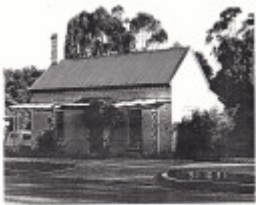
Brick House 88 Pitt St Eltham 1 - Shire of Eltham Heritage Study 1992
