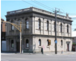
FORMER FREEMASONS HALL SOHE 2008
