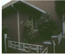
108 116 gladstone street south melbourne iron fence
