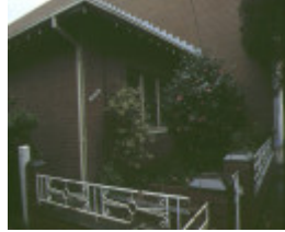
108 116 gladstone street south melbourne iron fence
