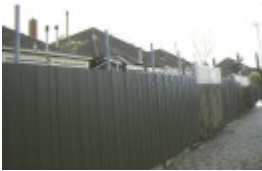
108 116 gladstone street south melbourne rear lane view
