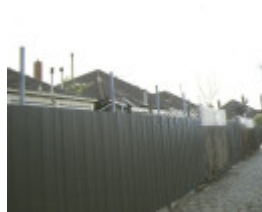
108 116 gladstone street south melbourne rear lane view
