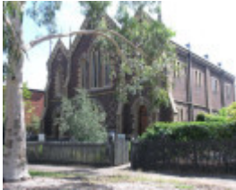
FORMER CONGREGATIONAL CHURCH SOHE 2008
