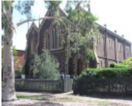
FORMER CONGREGATIONAL CHURCH SOHE 2008
