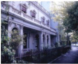
h00222 hazelwood terrace howe crescent south melbourne exterior from side she project 2003
