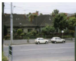
1 83 89 montague street south melbourne front view of row
