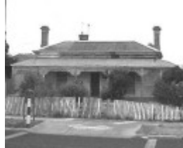
Site 093 - St Albans estate - 16 Arthur Street.jpg
