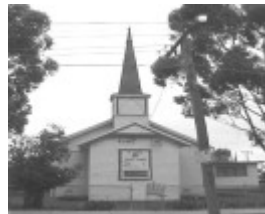
Site 094 - St Albans Uniting CHurch.jpg
